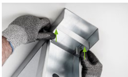
Figure 3: Raccordement coulissant au plafond
