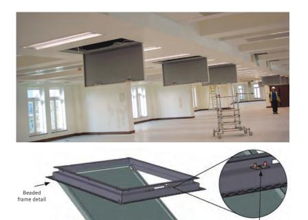
Unique tested interlocking design which prevents door opening in the event of fire
