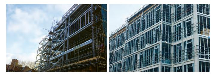
The Protektor SFS system is a widely recognised and proven method of creating external and internal stud frames across a wide and diverse range of construction projects.
