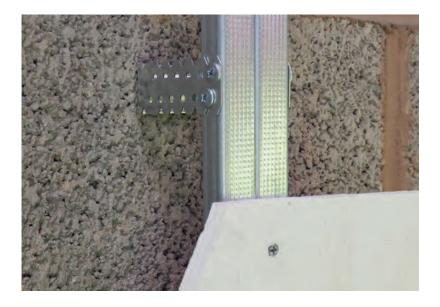
Protektor's Universal Lining system offers a fast, ideal solution for board applications to block/ brick wall constructions. The board layer is held away from the supporting wall with our brackets and profiles. The resulting cavity enables the contractor to run services behind the board layer.
