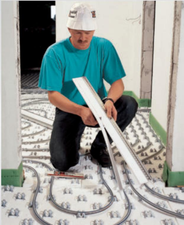
Trim the PE foam strip along the lower edge to the required height, according to the screed thickness. Mark and cut using an all-purpose blade.
